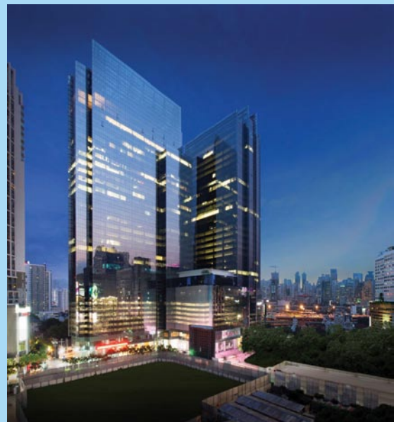
Picture of the Ninth Towers Grand Rama 9 Project
