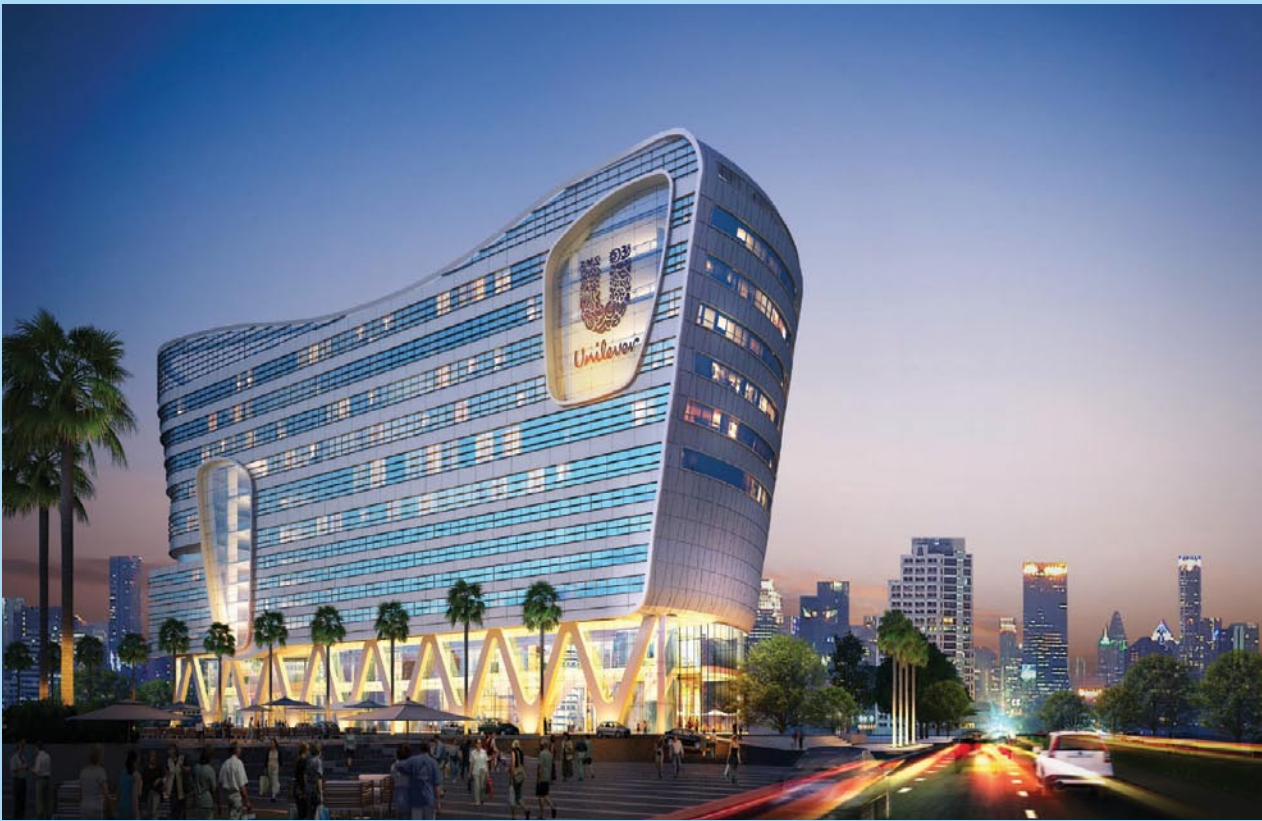
Picture of Unilever House Grand Rama 9 Project
